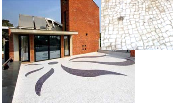
China Mosaic tiles installed on the roof
